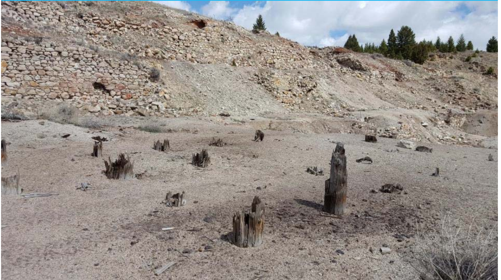
Supports for floor of leaching plant
