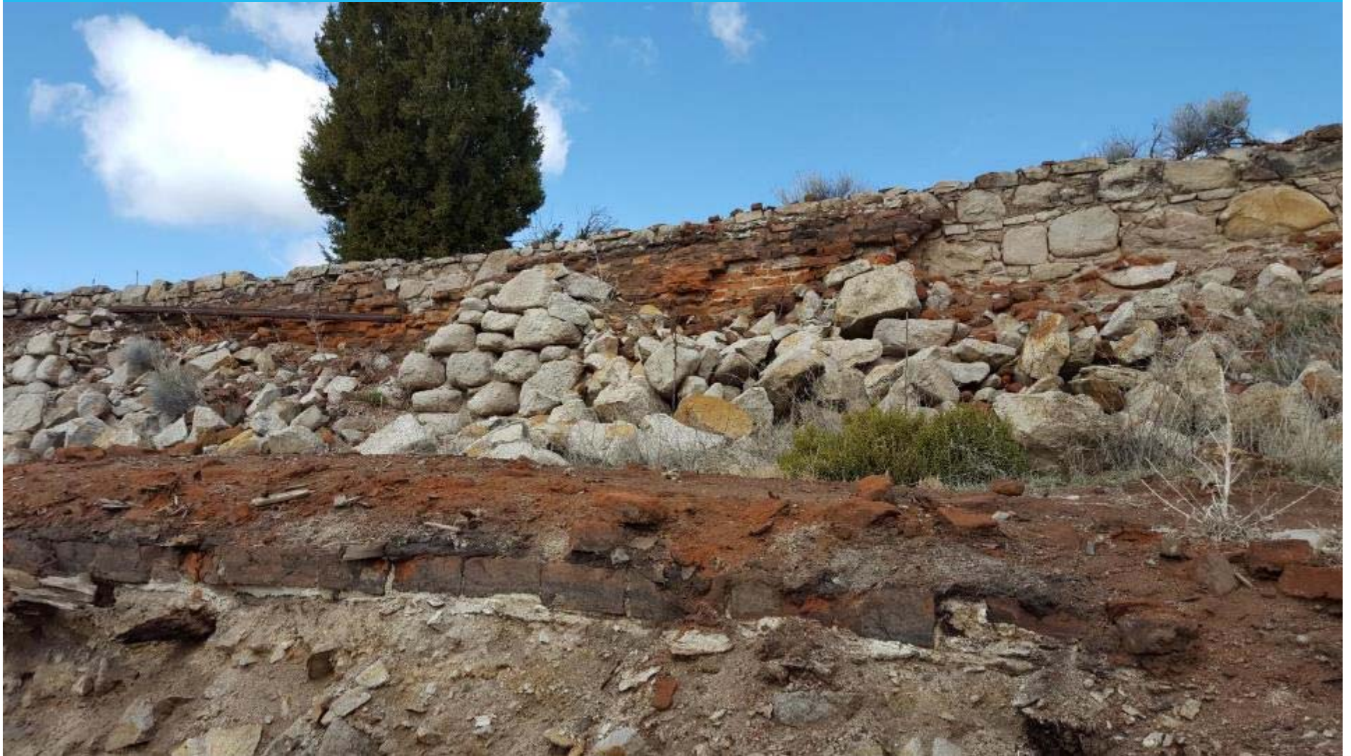
Cooling floor and general foundation
