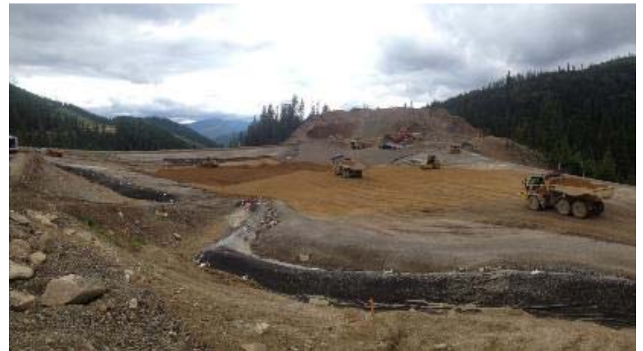
Prevent Run-On With Berms or Drainage Channels
