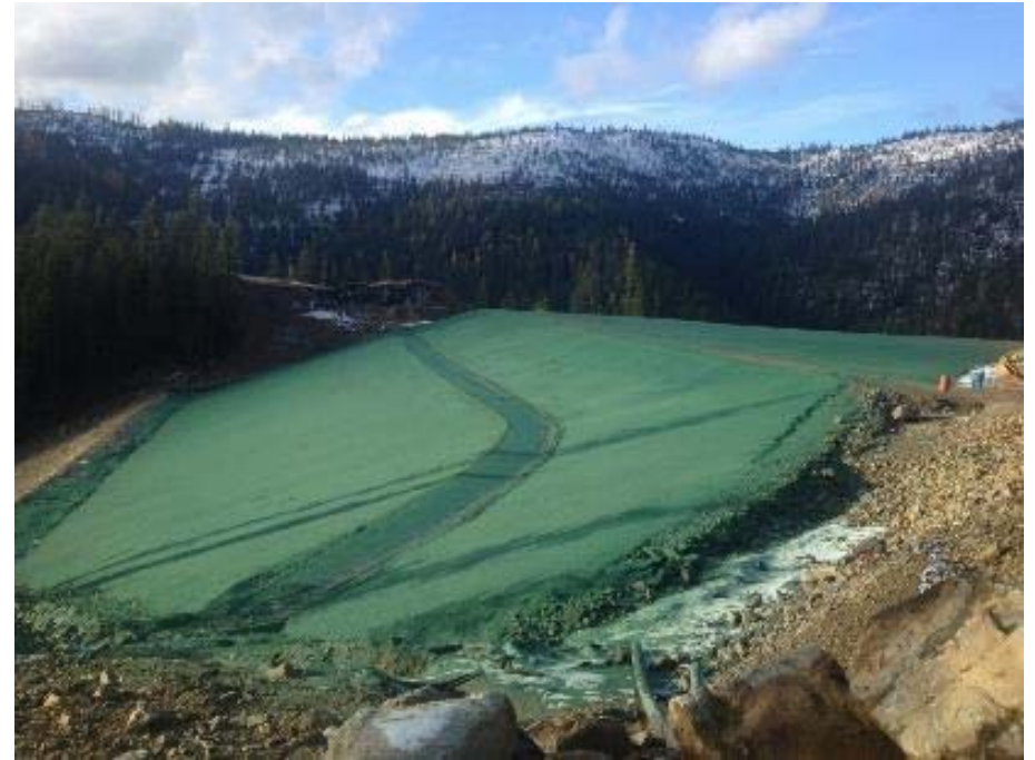
Temporary Stabilization for Temporary Covers – Bonded Fiber Matrix or Others
