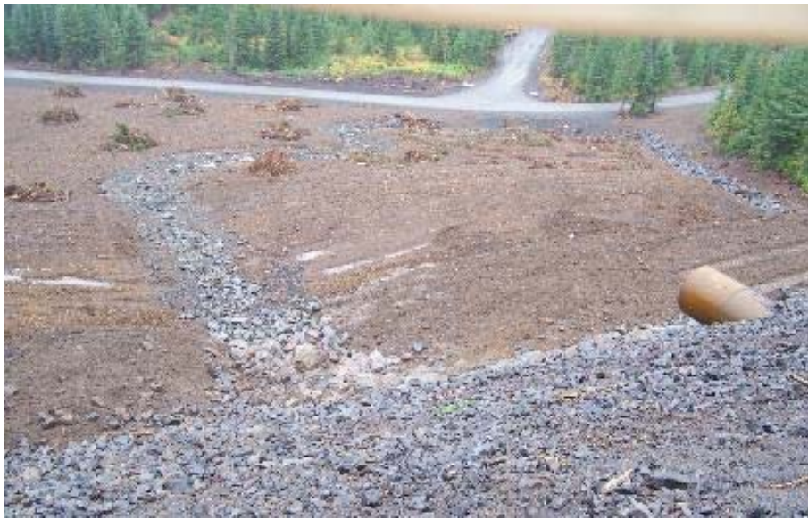
Controlled Run-On and Run-Off
