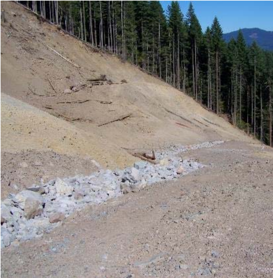
Run-On and Mid-Slope Run-off Channels
