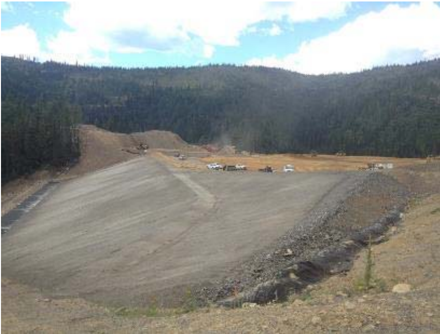
Reduce Slope Lengths with Mid-Slope Benches
